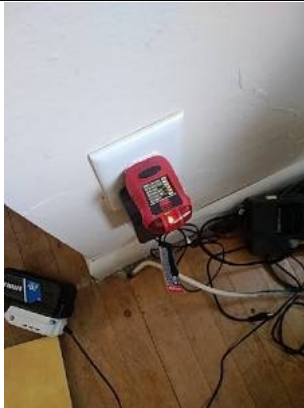
Example of open ground receptacles
