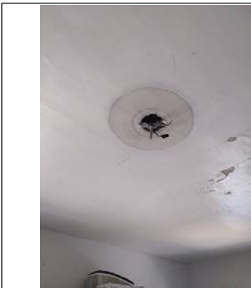
Open electrical termination
