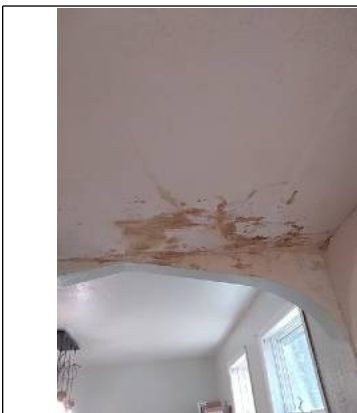
Moisture staining is present on the ceiling
