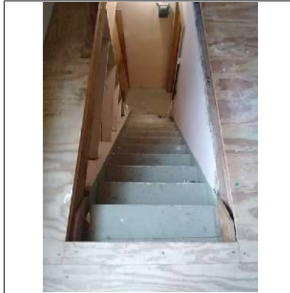
Recommend installing a handrail
