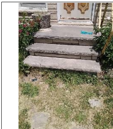
Front steps have uneven riser heights
