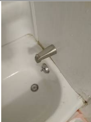
Nozzle is not secured
