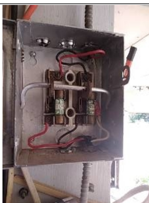
Double tapped circuits
