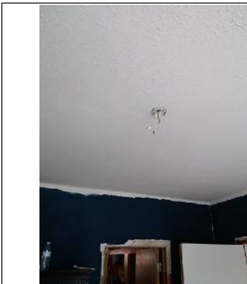
Open electrical termination
