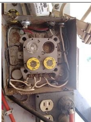
Sub panel 2-Missing fuse
