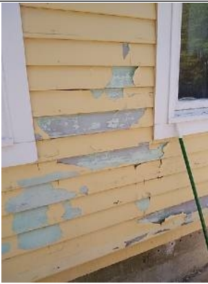
Example of peeling paint
