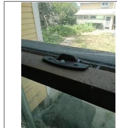
Missing window hardware
