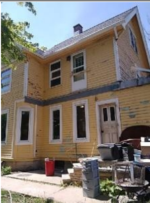
Example of peeling paint
