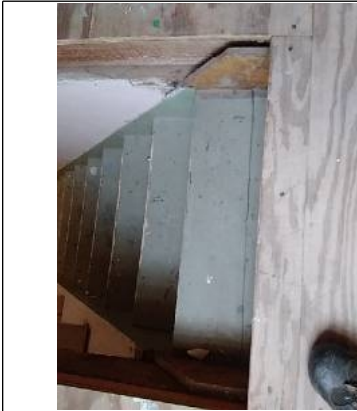
Cracked stair tread
