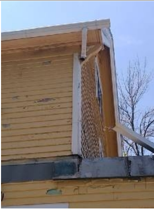
Example of where downspouts and extensions are recommended
