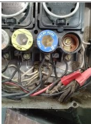
Double tapped circuits
