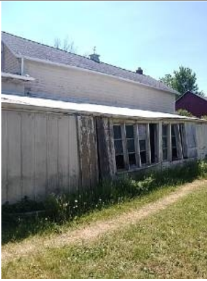
Example of improperly pitched gutters
