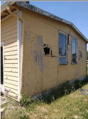
Example of damaged siding
